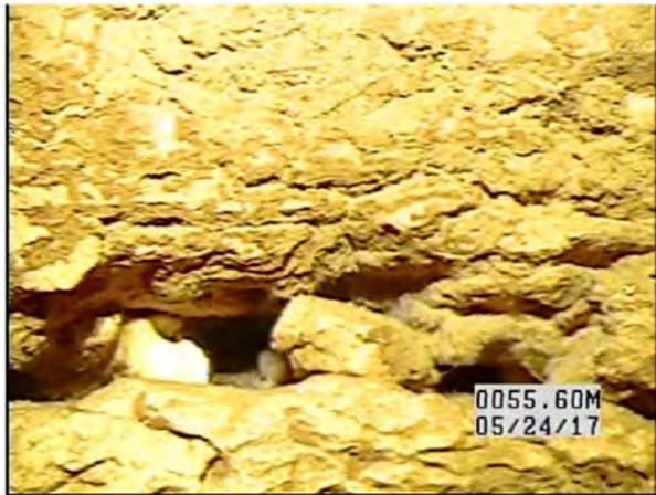
Photo 2: Side view of main water producing feature at 55.5m
